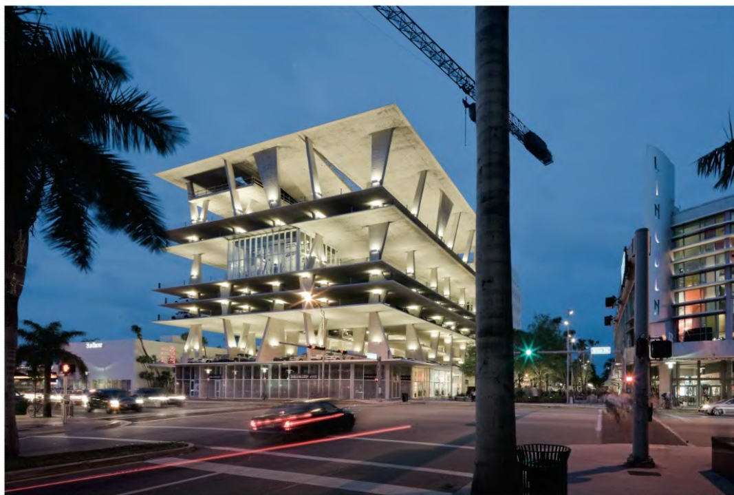
At 1111 Lincoln Road, the absence of exterior walls makes cars look as if they were perched on a cliff edge. Photograph by Iwan Baan.
